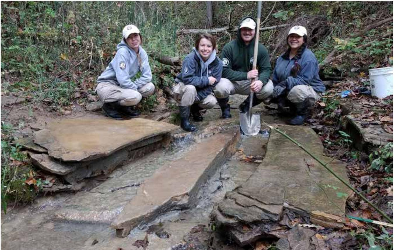
*The Arc's 2019 autumn AmeriCorps NCCC crew (one member short) proudly survey the completion of their cleverly engineered bridge—constructed solely with natural stone leveraged from the site and anchored together with hydraulic cement. The new bridge lies on the God's Country I tract and will one day be part of a new Sanctuary hiking trail that God's Country II's acquisition will make possible.*
