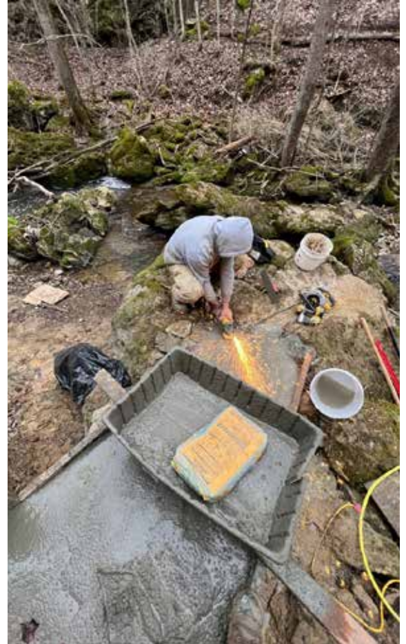
Top photo left page: Endurable sandstone slab steps were constructed at Saltpeter Cave at the Honeycomb Rocks Preserve from locally collected materials. Top Left: Land Manager Ethan King ponders how to overcome the challenge of the creek crossing presented at Quiverheart Gorge Preserve. Top right: Ethan King is hard at work cutting rebar and pouring a cement walkway that will anchor the bridge which is in the process of being built. All three photos were taken by Tim Pohlar, Arc Land Manager and Ethan's colleague.
