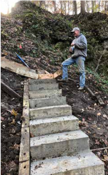
TOP LEFT: Craftsman David Conley constructing 80 concrete steps on the Barrett's Rim Trail to navigate its dauntingly steep descent into the Rocky Fork Gorge. MIDDLE: Sandstone stepping stones carry hikers across a wet spot at Rock Run Preserve. RIGHT: The crew constructed a staircase at Quiverheart Gorge Preserve using century-plus old beams that were recycled from a deteriorating mill house at the Highlands Nature Sanctuary. All photos by Tim Pohlar.
