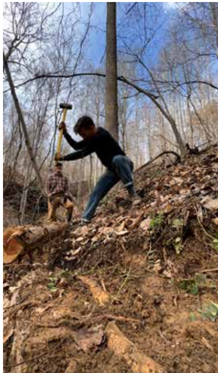
ABOVE LEFT: Arc Land Manager Elijah Crabtree drives rebar anchors trailside at Ohio Hanging Rock Preserve. Photo by Tim Pohlar. MIDDLE: Land Manager Tim Pohlar sits on a metal beam support for a new bridge. The beam was recycled from an abandoned house trailer. Photo by Ethan King. RIGHT: Stewardship Staff Sam James and Tim Pohlar perform the final touch by erecting signs at the newly opened trail system at the Arc's Kamama Prairie Preserve. Photo by Elijah Crabtree.
