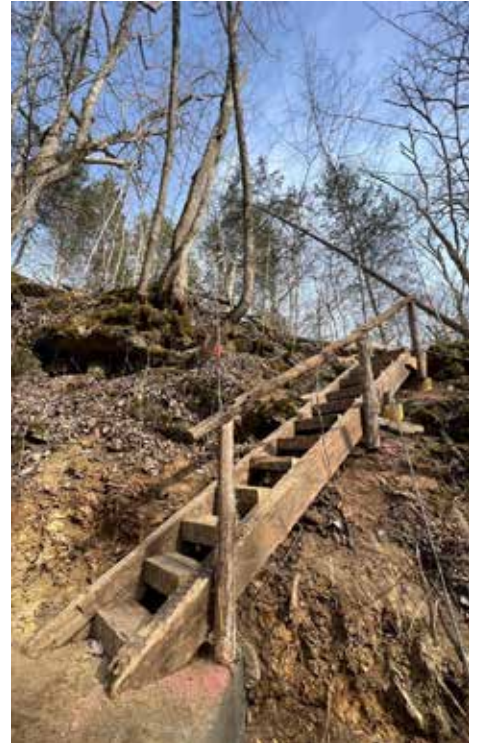
TOP LEFT: Craftsman David Conley constructing 80 concrete steps on the Barrett's Rim Trail to navigate its dauntingly steep descent into the Rocky Fork Gorge. MIDDLE: Sandstone stepping stones carry hikers across a wet spot at Rock Run Preserve. RIGHT: The crew constructed a staircase at Quiverheart Gorge Preserve using century-plus old beams that were recycled from a deteriorating mill house at the Highlands Nature Sanctuary. All photos by Tim Pohlar.
